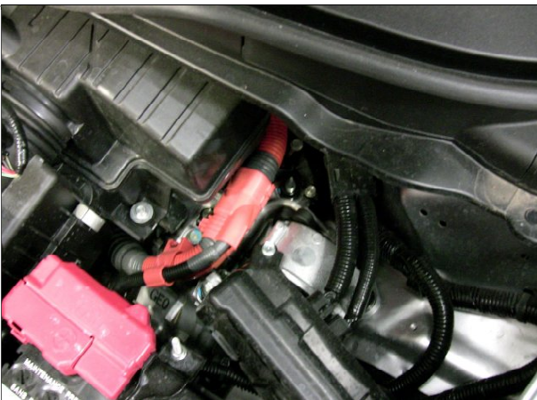
Figure 9 / High voltage cables are always orange
